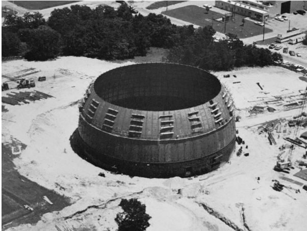
Fig. 1. Brookhaven's High Flux Beam Reactor (HFBR) containment vessel under construction, June 1962. Credit: Department of Energy, Brookhaven National Laboratory.
