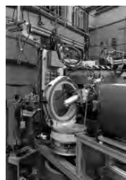
Figure 17: New four-circle neutron diffractometer 4C 1992 at reactor SAPHIR.
