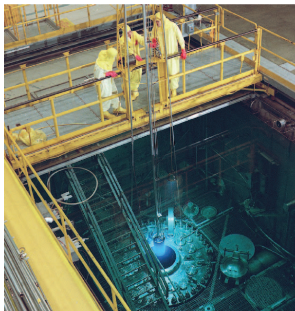
Figure 7. The High Flux Isotope Reactor achieved criticality in August 1965. HFIR is designed to produce super heavy elements such as californium, and its intense neutron beams also are applied to materials studies. HFIR became a user facility when the National Center for Small-Angle Scattering Research opened in 1980, and continues to operate today. Image courtesy of ORNL.
