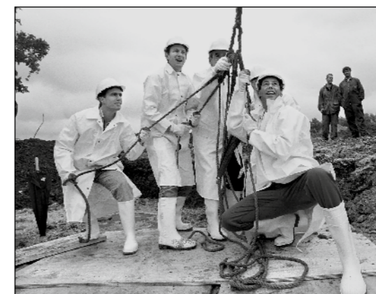
2001, 2 October. Tim van der Hagen drives the first pile for the new office building
