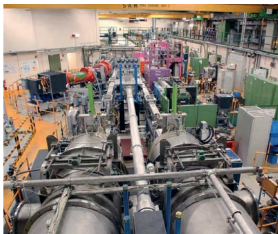
| View into the ELLA hall at DIDO with its suite of small-angle cameras (Copyright JCNS, FZ Jülich).
