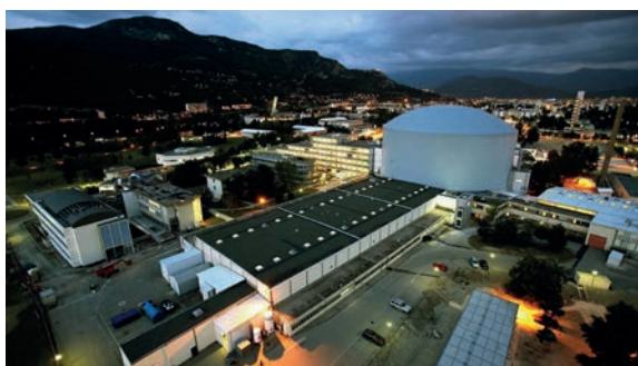
View on reactor, administrative building and neutron guide hall of the ILL at Grenoble (Copyright ILL).
