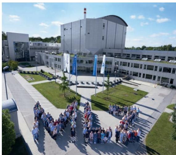
Heinz Maier-Leibnitz Zentrum (MLZ), a cooperation between FZ Jülich, HZG, TUM, MPI and further 10 university groups for the scientific use of the FRM II (Copyright: Schürmann/ TUM).
